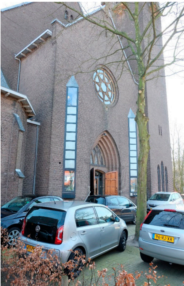
Figure 5 Providing a sufficient number of parking lots is an important question in the re-utilisation of churches (case 14) Photo: authors
